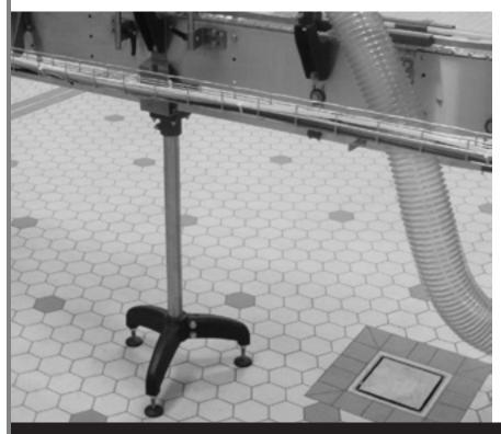
**KAGETEC** provides chemical resistant, hygienic, industrial flooring systems consisting of slipresistant ceramic tile and integrated stainless steel drains.
